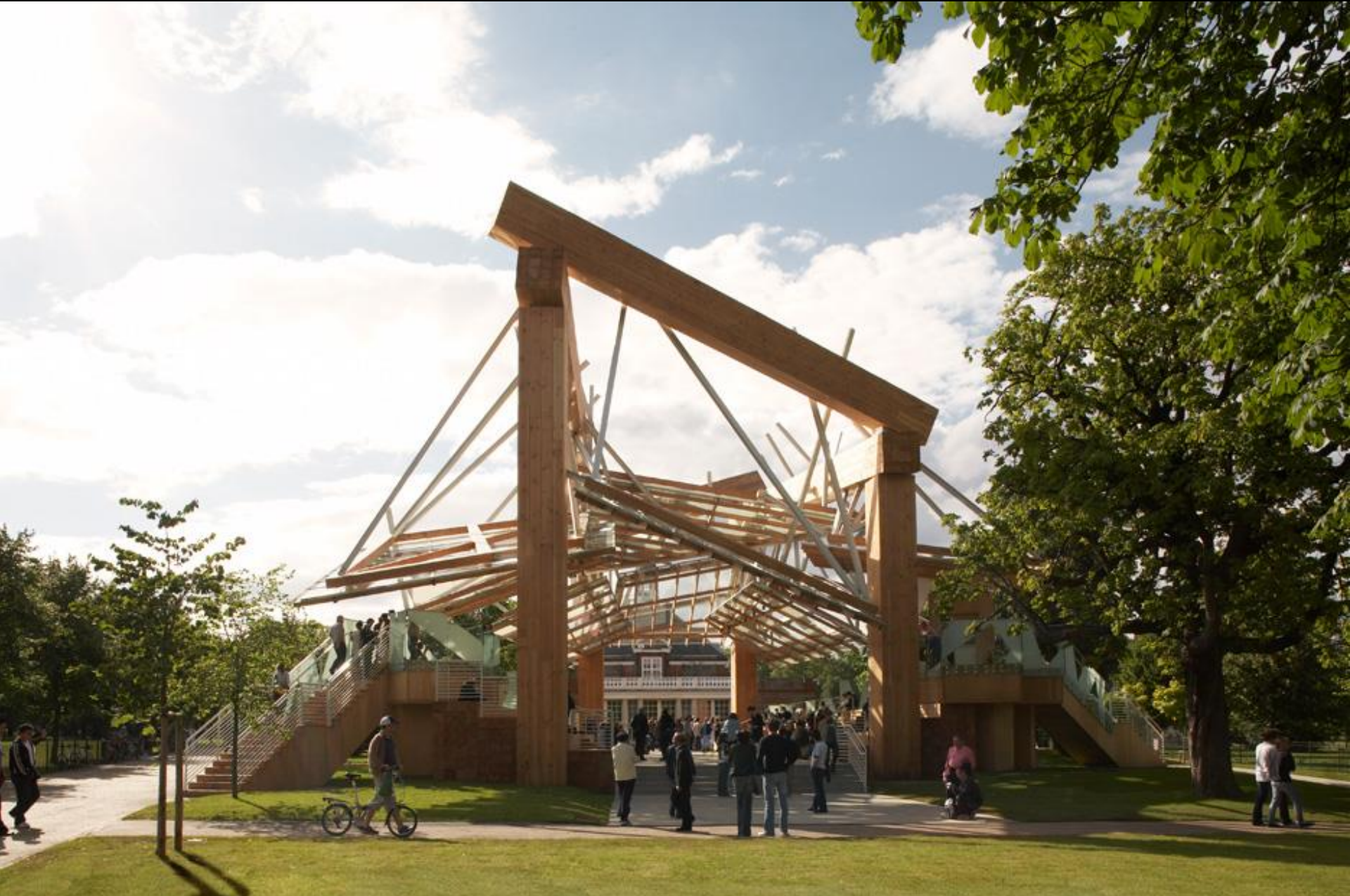
Frank Gehry's 2008 Serpentine Gallery Pavilion consisted of four wood-clad steel columns, which supported a series of large timber planks and beams.
